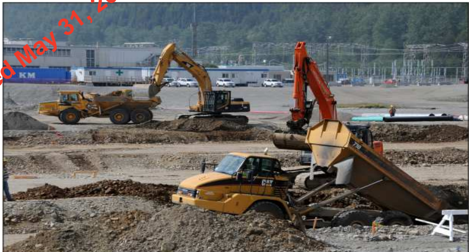
Kitimat Modernization Project - June 1, 2010 Anode Pallet Storage Building - Foundation preparation work
