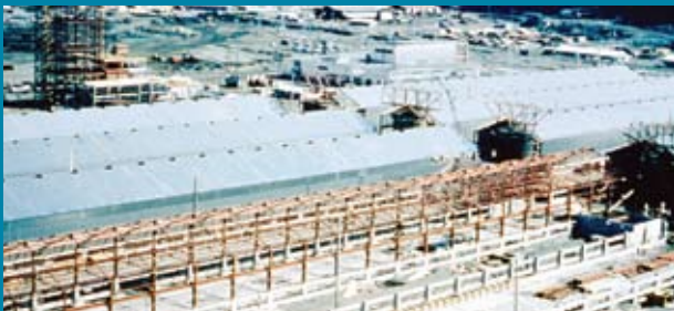
An aerial view of unfinished pot lines. (at left)
